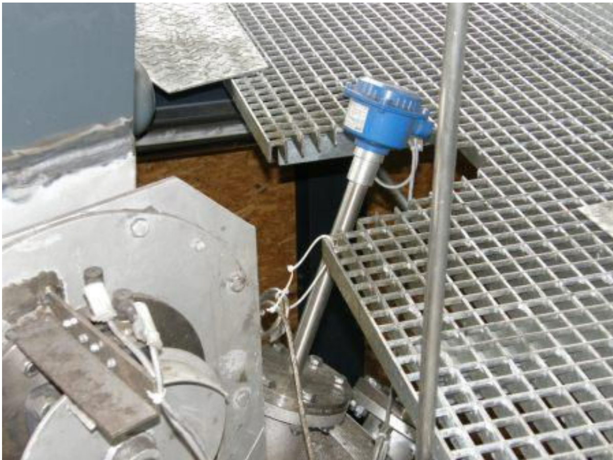
One of the two ROTONIVO 6000 level limit paddle switches supplied by UWT
