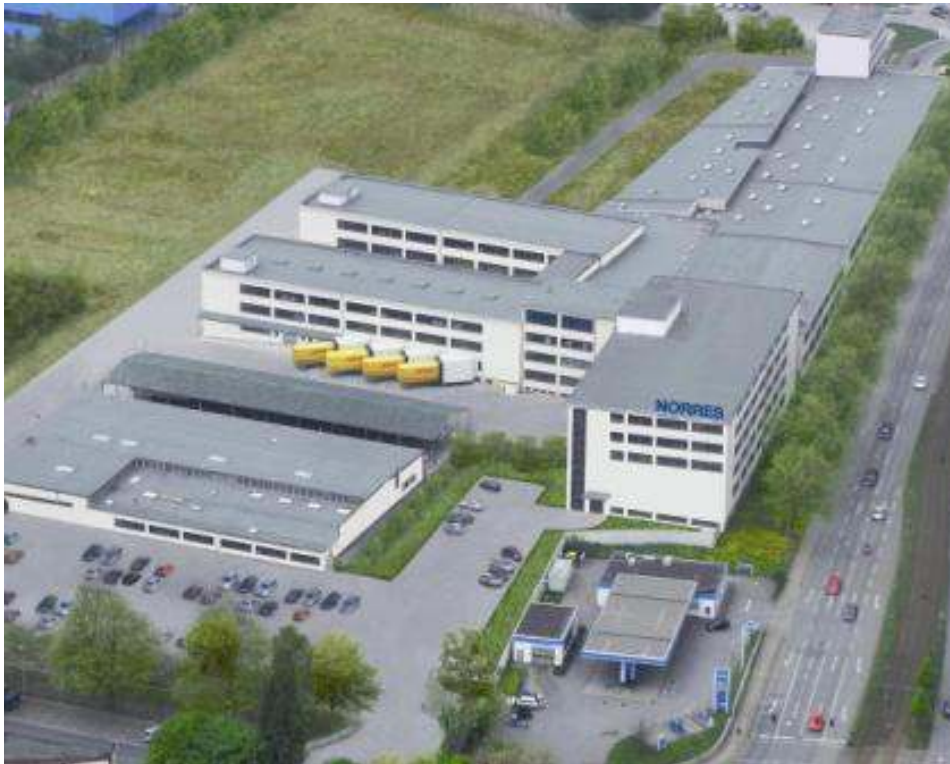
Norres' new larger and fully integrated headquarters
