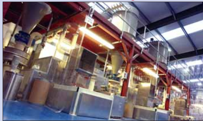
British Rema's Chesterfield toll processing facility.
