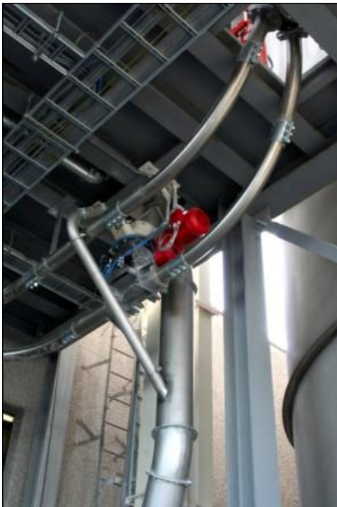
Installation of Dinnissen Slow Flow Conveying system
