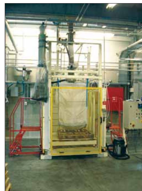
Spiroflow bulk bag filling rig at Nanocyl showing bag suspended ready for filling with safety cage closed; unprecedented levels of filling accuracy are attained.
