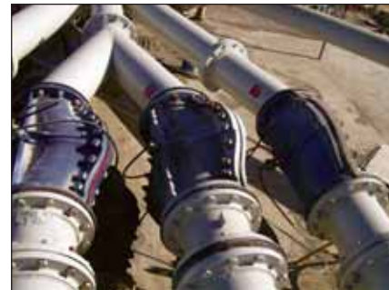
Linatex pneumatic pinch valves installed on delivery lines conveying cement powder to storage silos. The valves are very well suited to high frequencies of opening and closing, added to which the premium rubber liners protect against abrasion damage and their low-friction properties prevent risk of blockage.
