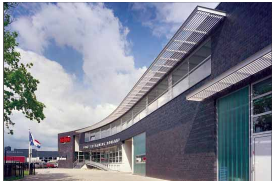
The Chronos BTH headquarters at Eersel, the Netherlands, houses administrative offices, a test plant and extensive state-of-the-art manufacturing facilities.
