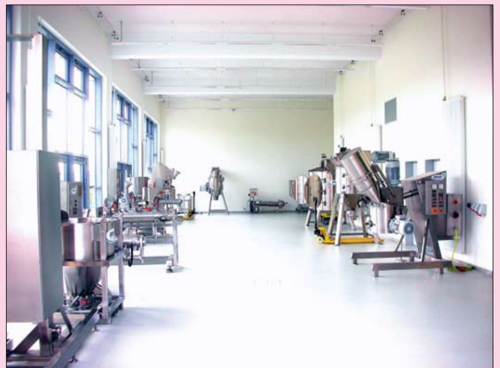
View inside amixon's Paderborn test plant.
